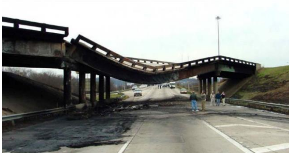
Fig. 4 Failure of I-65 bridge (courtesy of ALDOT)
