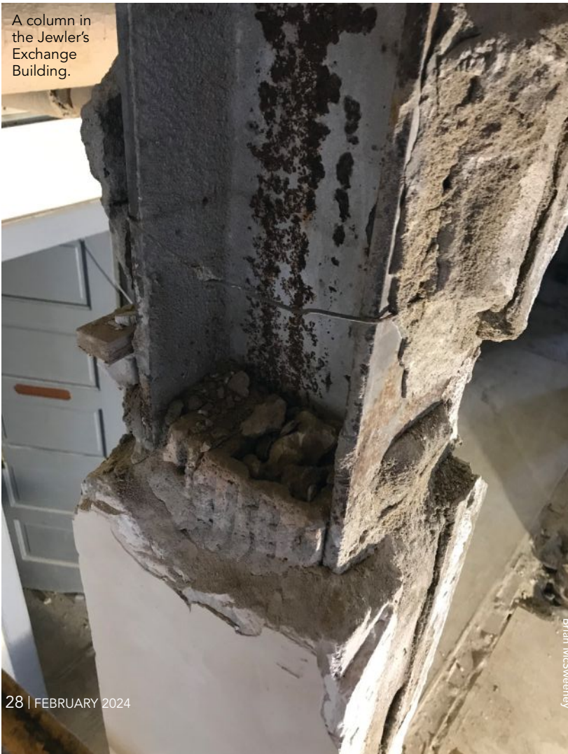
An original connection in the Jeweler's Exchange Building
