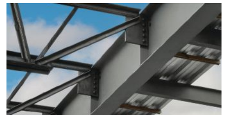
Joist reaction point occurs at beam centerline
