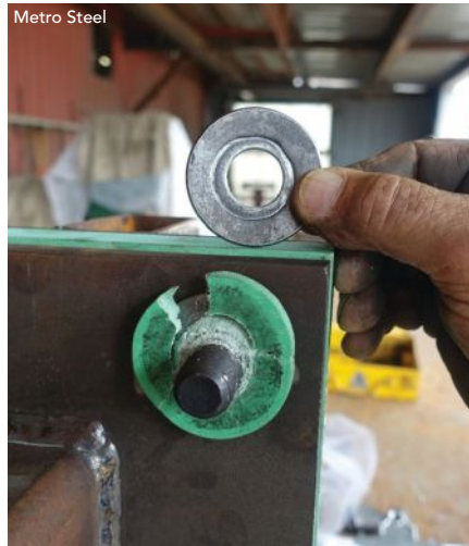
Fig. 6. Thermal washer failure at bolt with regular oversized washer.
