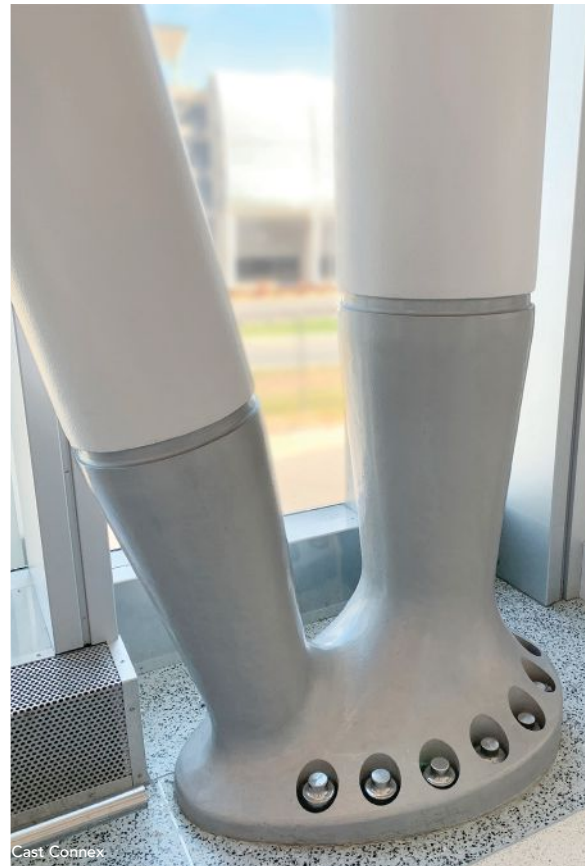
above: Two examples of architecturally exposed steel castings: nodes are used in the diagrid tower at The Leaf at Assiniboine Park in Winnipeg, Manitoba (left) and V-column bases are used at Charlotte-Douglas International Airport (right).
