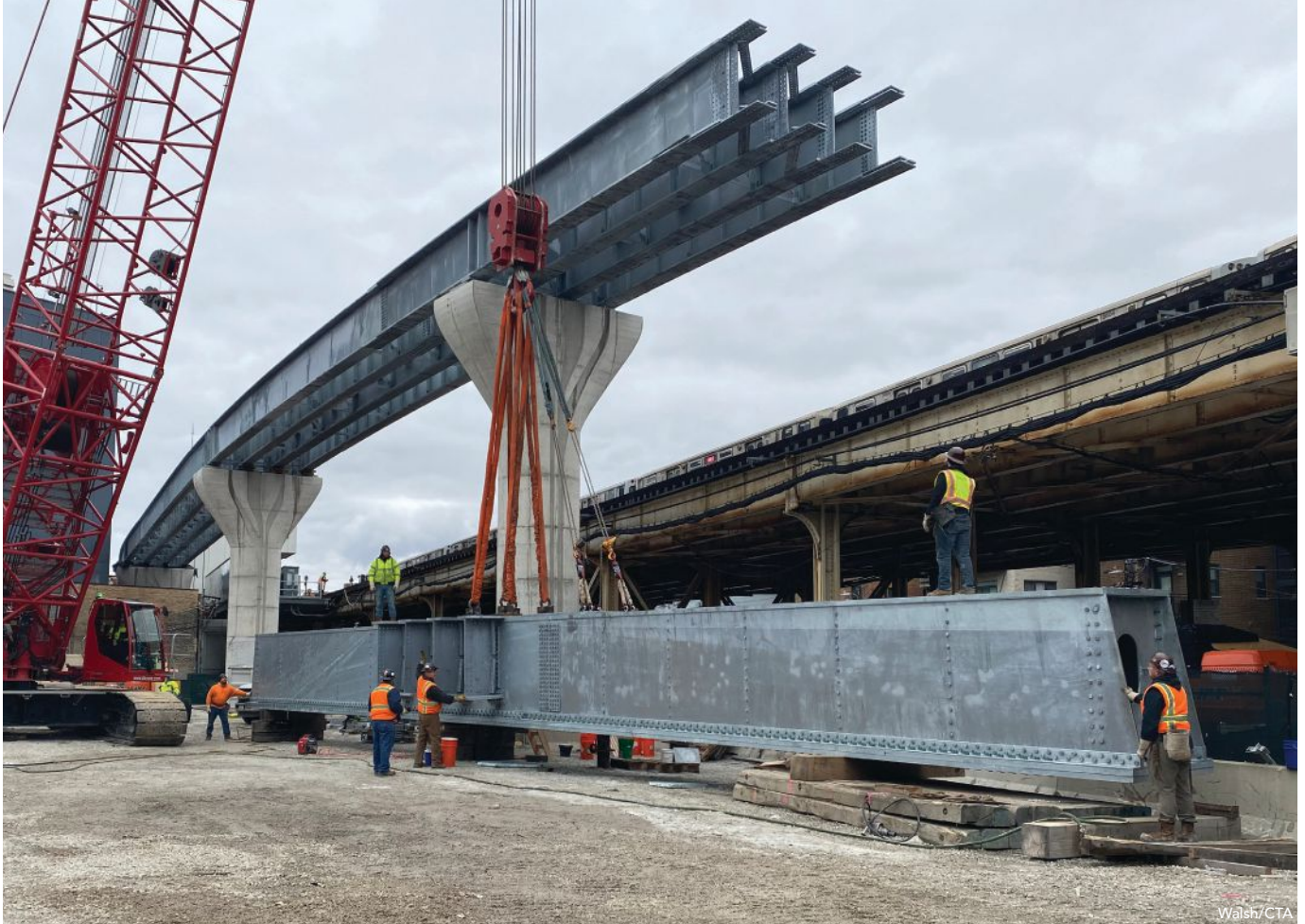
above: The flyover girders and straddle beam being erected.
